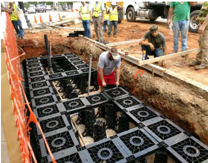
Above: Plan detail for Harrison Avenue. Left: Soil cells under construction for street trees in Thomasville, GA; structural soils support tree health and longevity, stormwater retention, treatment and cleaning.
